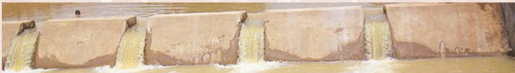
Masonry Check Dam
