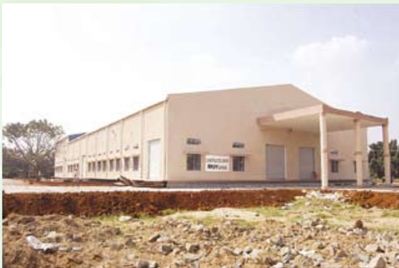
New Godown Constructed at A.P.S.S.D.C. Ltd., Srikalahasthi
