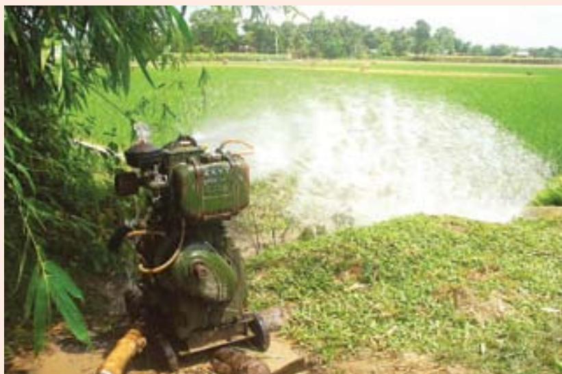
A Shallow Tube Well with Diesel Pump Set supported under RKVY irrigating Paddy in Nagoan District of Assam
