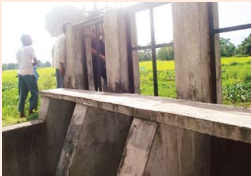
Christian Basti Flow Irrigation Project (Local Name: Kritupal Bheta), Christian Basti, Sonitpur
