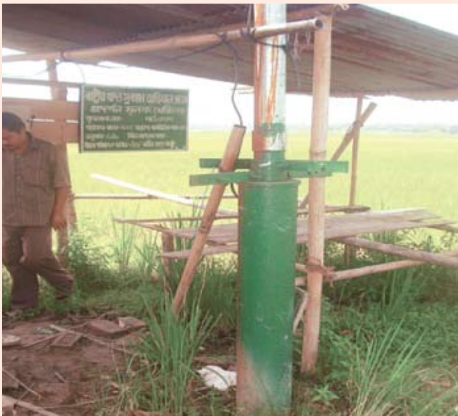
A Deep Tube Well at Hebeda Village. The beneficiary Farm Management Society subsequently received assistance under NFSM for Rice Demonstration
