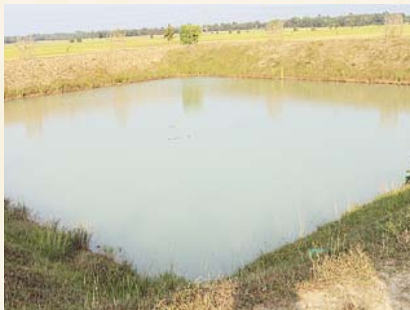
Micro Irrigation Tank
